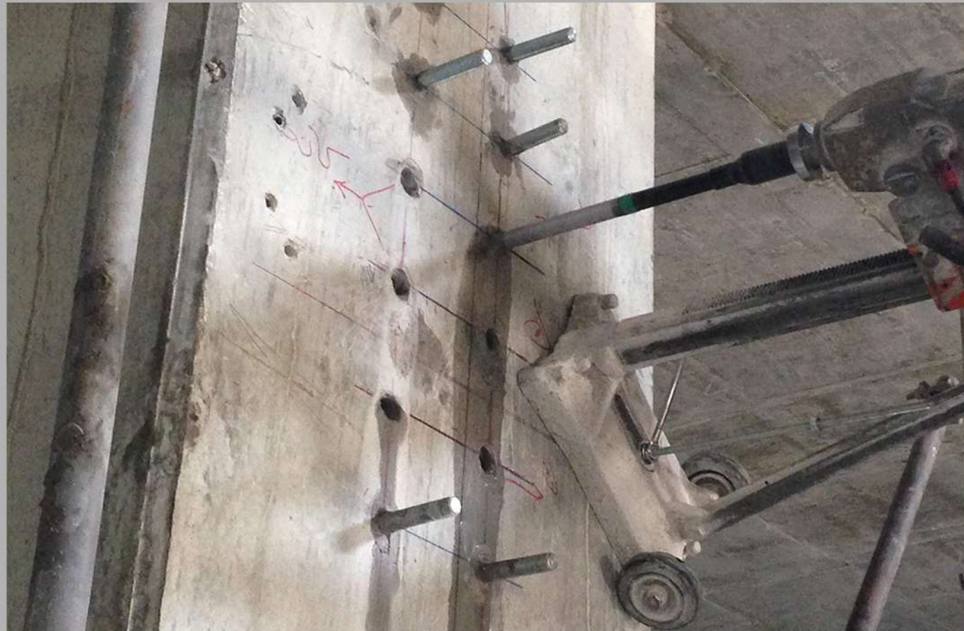
CORE DRILLING WITH ANCHOR BOLTS
