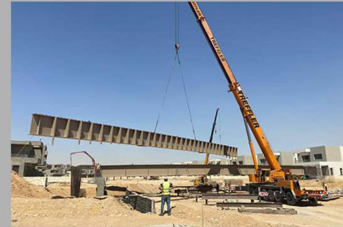
ASSEMBLY AND ERECTION
